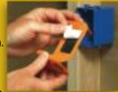
new-work box to indicate the size and location of the opening needed in the drywall. The low-voltage bracket may be left in place when installing the MIW-POWER.
